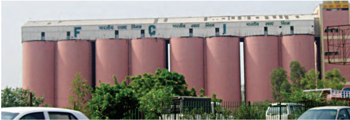
Fig. 1.10 (a) : Silos for storage of grains
