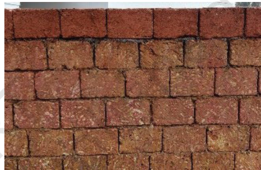
Fig. 11.7: Laterite rocks used as bricks
